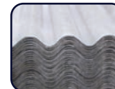
Asbestos and concrete containing sheets – slate
