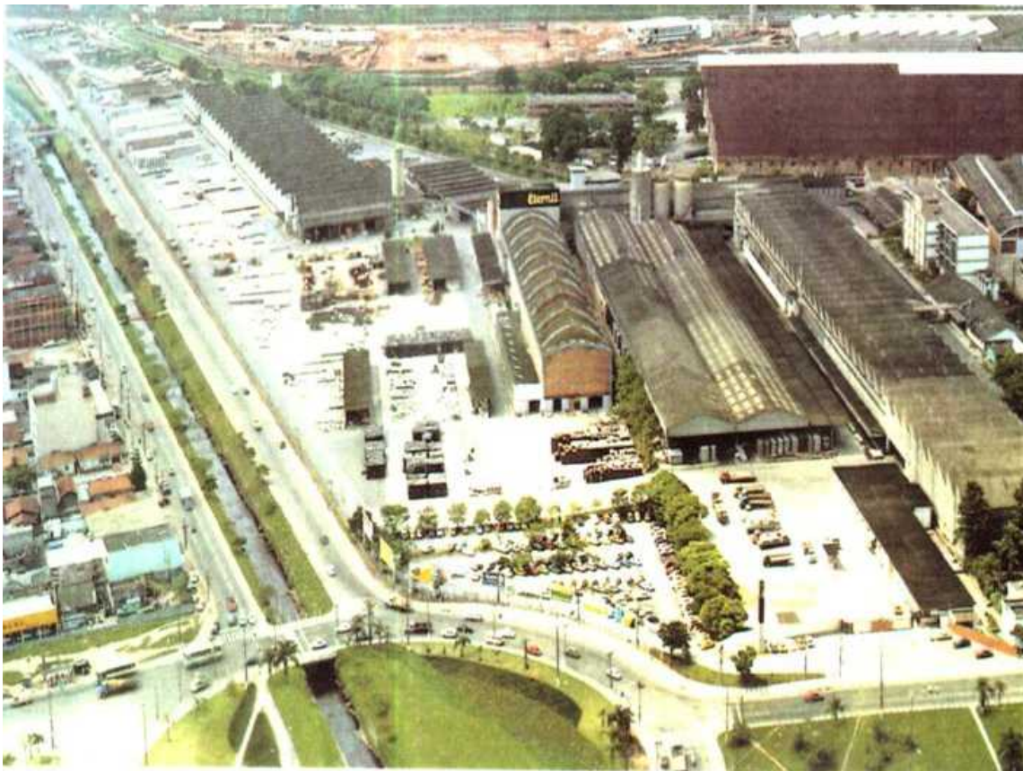
The Osasco Eternit plant as it was at the time of its closure in 1993. Photo: Eternit periodical "O Telhadinho."
