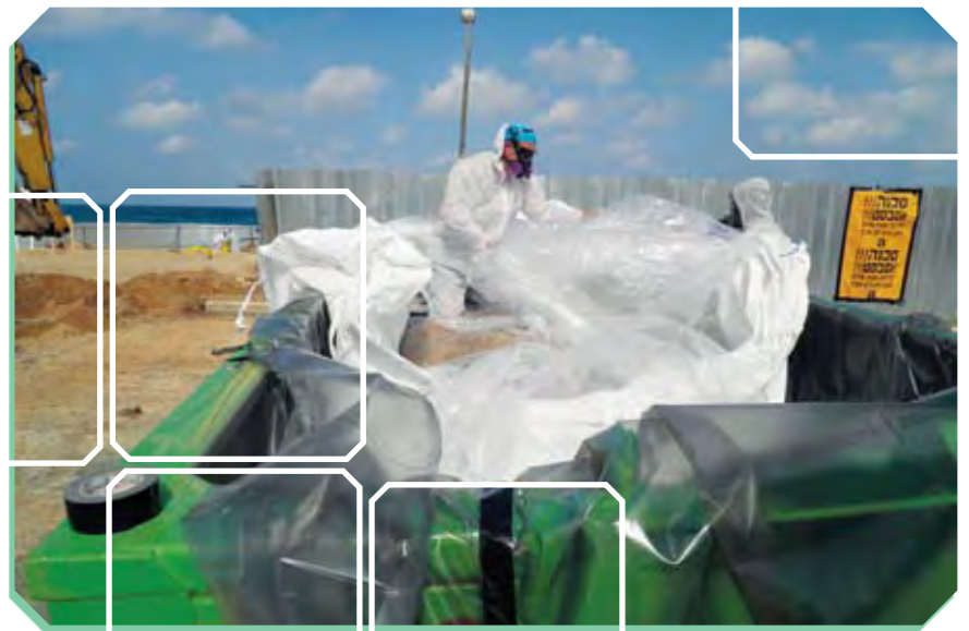
Packing asbestos for removal / Photo: Yoram Varga
