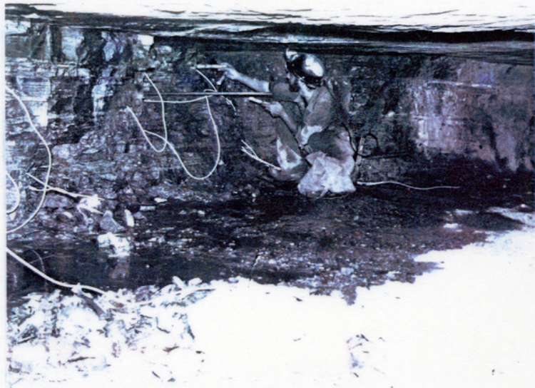
WITTENOOM ASBESTOS MINER MINING IN STOPE - 38 INCH HEIGHT
