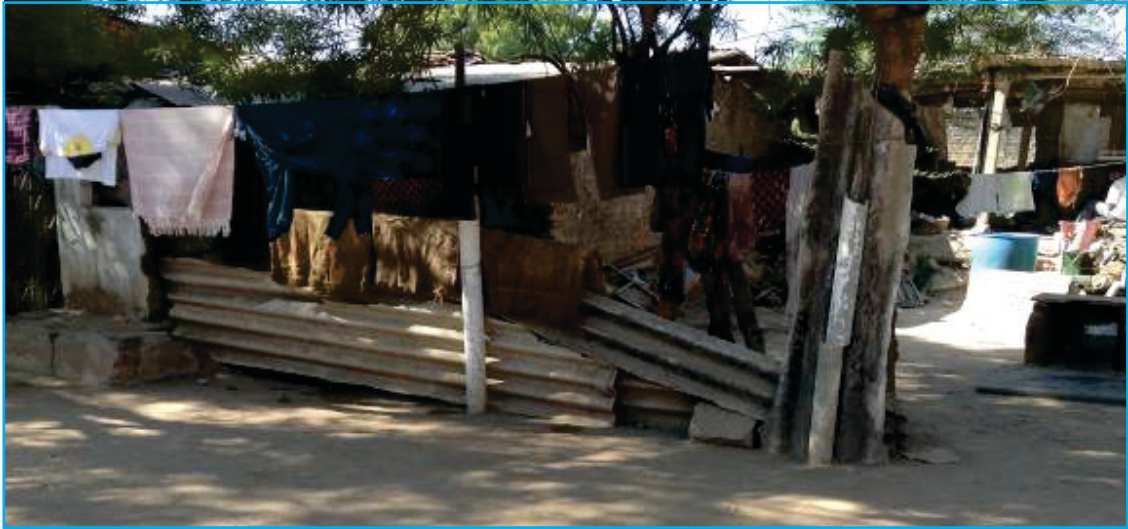
Figure 10: Asbestos Cement Sheets in low-cost housing
