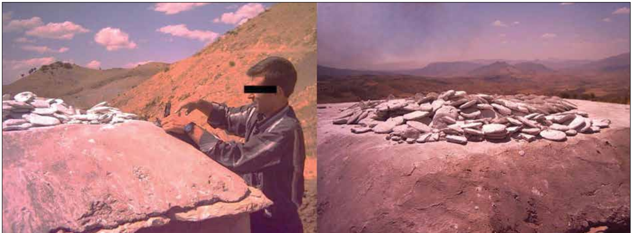
Figure 8. The white soil is laid on the roofs for drying. It will be used when necessary. Pay attention to the roof cover. A typical example of white soil cover (The archive of Dr. A. Şenyiğit)
