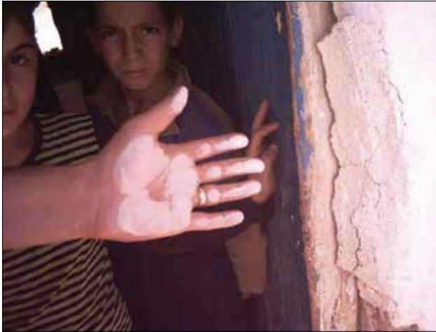
Figure 11. White soil plastered on the wall easily adheres to the existing material (The archive of Dr. A. Şenyiğit)
