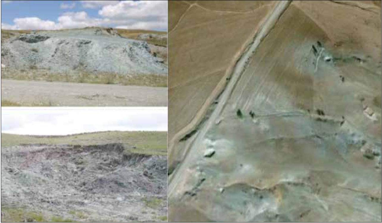
Figure 2. Mounds with natural asbestos near the roads in Sivas (The archive of Dr. M. Bayram)
