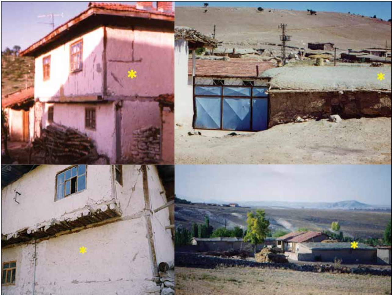
Figure 9. Houses with white soil plastered walls and covered with white soil roofing (The archive of Dr. M. Metintaş)
